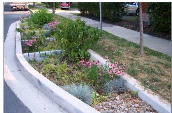
Figure 53: Example of a rain garden built into the sidewalk
