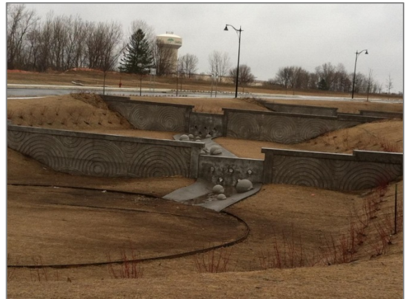
Figure 54: Tartan Crossing's artful stormwater design
