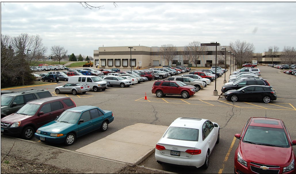
Fig. 1: View looking east towards the SuperValu headquarters.
