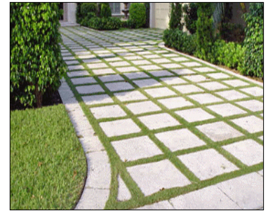
Fig. 43: Pervious driveway/walkway. Image courtesy of: reimaginingcleveland.org
