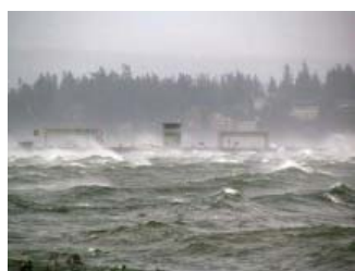
Top: 520 bridge mid-span during windstorm
