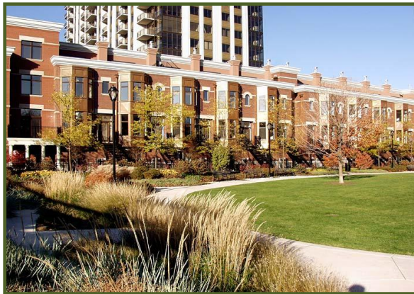
Figure 15: South Bryn Mawr residents did not appear to favor wide expanses of lawn
